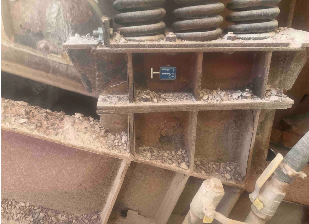
Structure Test RH FE 10/20/2022 10:25:43
