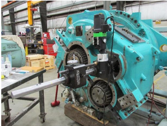
Fig. 3 Shop application of gearbox repair method
